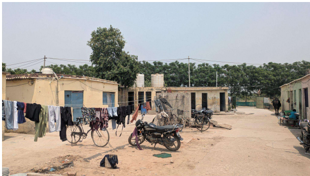
Figure 3: A single-storey Vehra with asbestos roofing with 12 rental units
