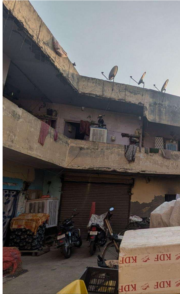
Figure 6: A four-storey Vehra
