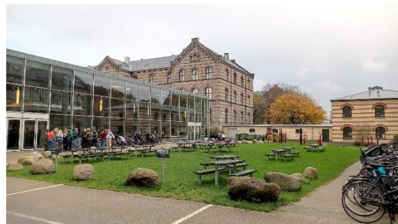
Figure 19: Yard 3, view towards building 34. From west to east. Source: Author
