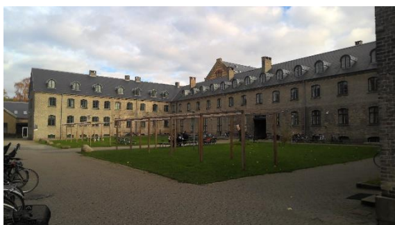
Figure 18: Yard 5, view towards eastern courtyard corner. Source: Author.
