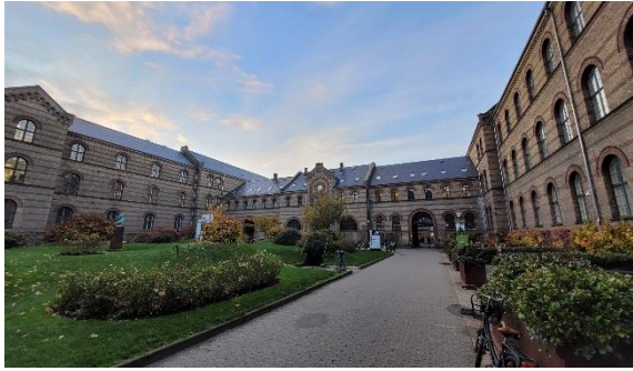
Figure 14: Yard 1, view towards building 01. Source: Author
