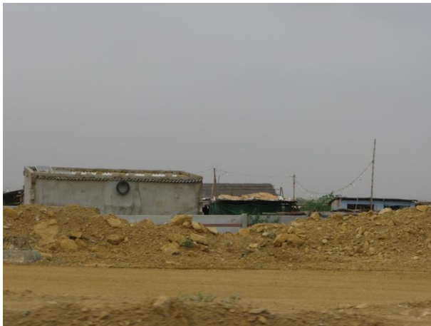
Figure 4 (Author, 2024) Construction residue towering over ADG village wall.
