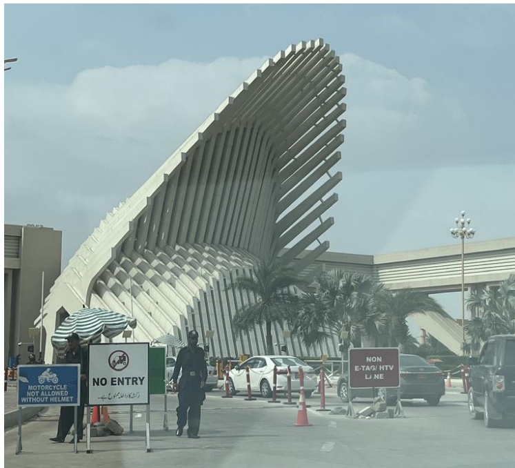
Figure 9 (Author, 2024) BTK main gate and its security apparatus. Signs barring entry of rickshaws and motorcyclists without helmets are abundant along with surveillance cameras, barricades and armed guards patrolling the entrance.
