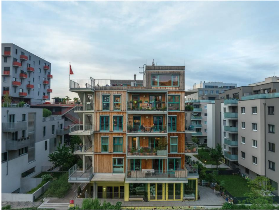
Gleis21, a co-housing project in Vienna. Luca Locatelli for The New York Times
