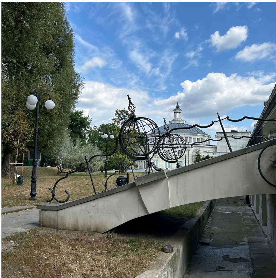
Fig. 14: Balustrade of the stairs to the Community Cultural Centre (Dom Kultury) at the WSM, with the Comedy Theatre in the Background.
