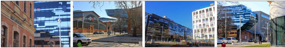
Figure 23. Architectural mix in Neumarx
